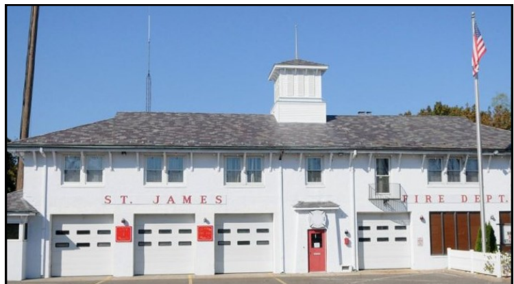
St. James Firehouse Route 25A
